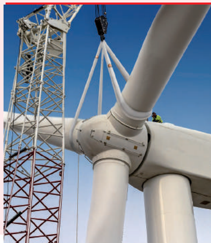
UHMWPE fibre slings up to 2100 tons mbl
