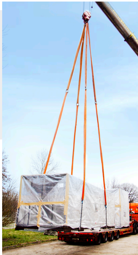
Lifting with chains combined with round slings
