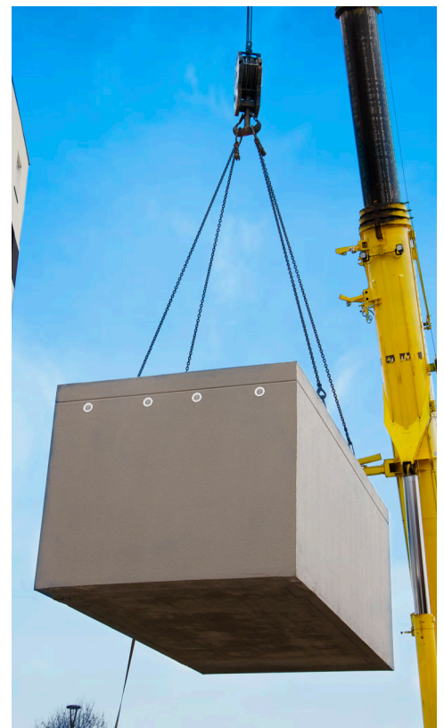
Lifting with chains only.
