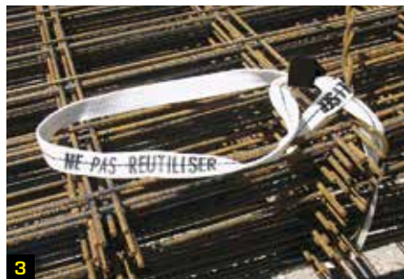
3 The system is in place and operational.
