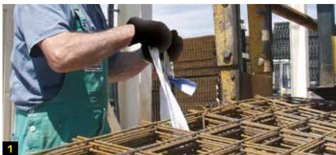
1 Pass the sling through the mesh of the welded mesh. Pass the hook end of the sling through the loop. Thread the sling into the Li-1 plastic part, observing the direction of the arrow on the housing.
